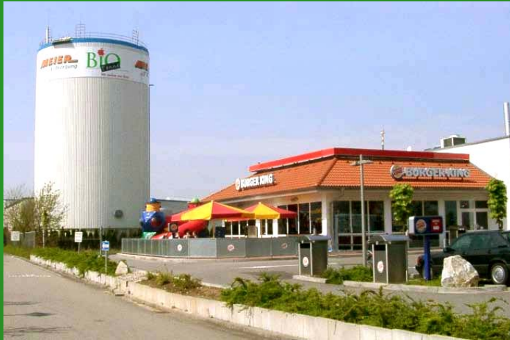
Food waste digester in Europe
