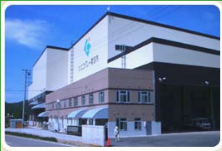
Gasification facility in Japan
