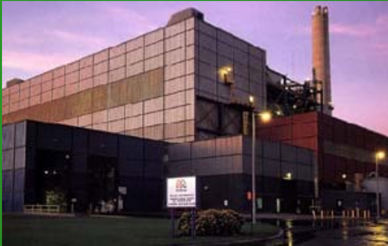
Southeast Refuse Recovery Facility (Long Beach, CA)
