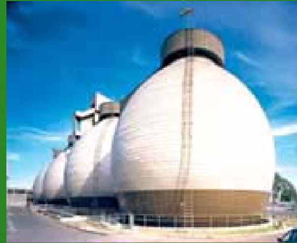
Biosolids digesters at LA's Terminal Island Wastewater Treatment Plant
