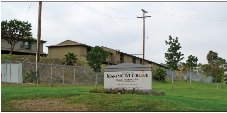
Marymount College's plans call for new classrooms, residential, dining and recreational facilities at their Palos Verdes Drive North location.
