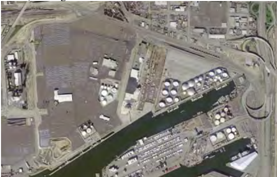
Aerial view of Pier B
