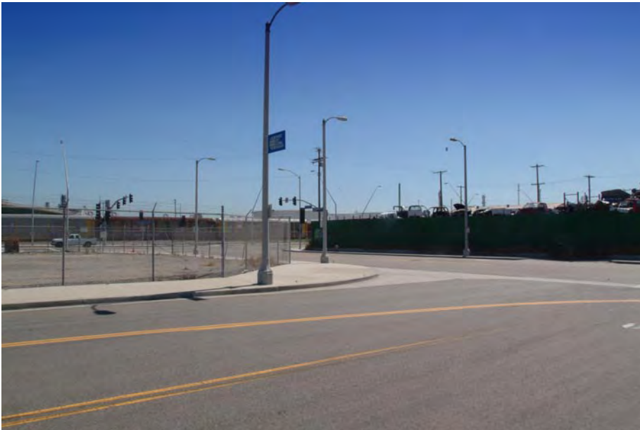
Anaheim Way, at Farragut, looking southwest
