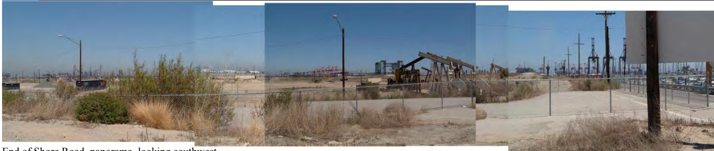
End of Shore Road, panorama, looking southwest
