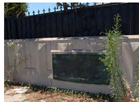
Gaffey Street Bridge
