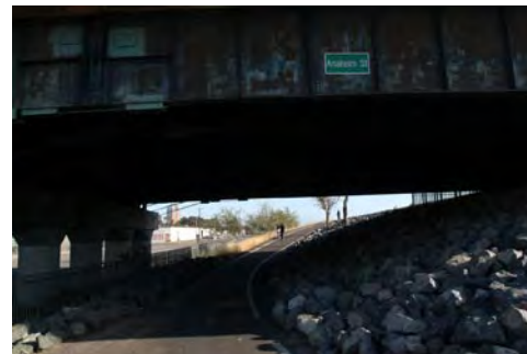
Bike path under Anaheim Street Bridge
