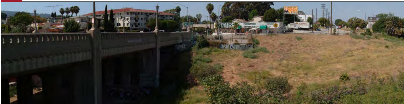
Gaffey Street Bridge
