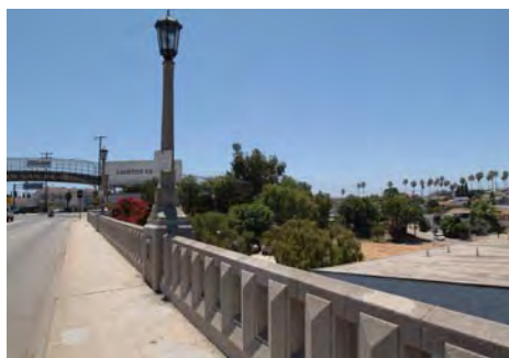
Gaffey Street Bridge
