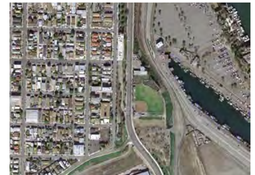
Aerial view of Gulch Road
