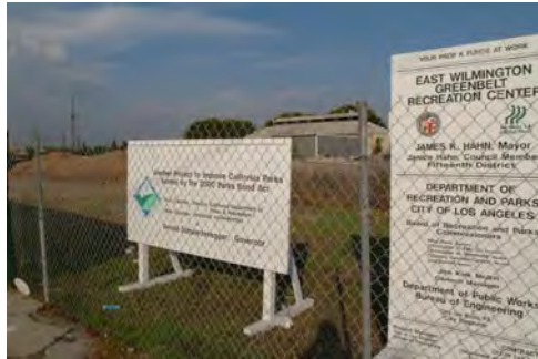
Site of future Recreation Center
