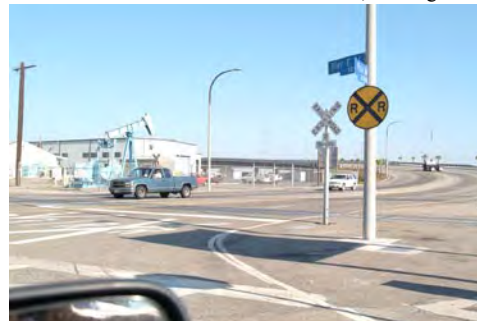
Pico at Pier E, looking south
