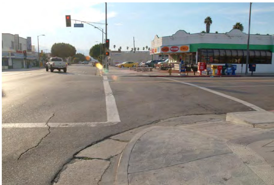
Anaheim at Broad, looking west
