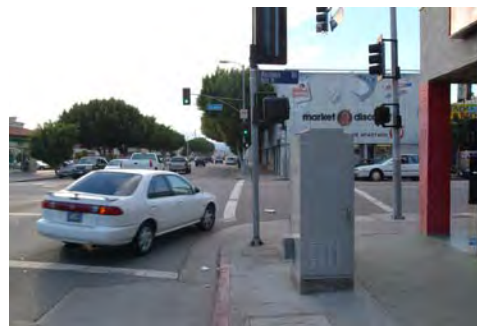
Anaheim at Avalon, looking west
