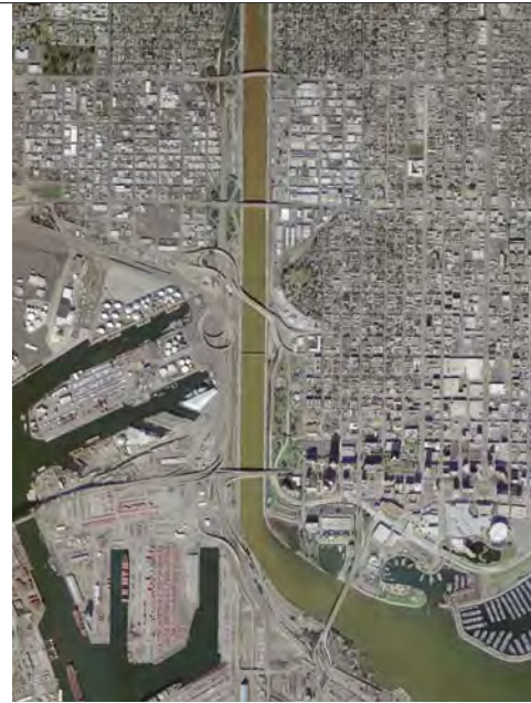
Aerial view of L.A. River
