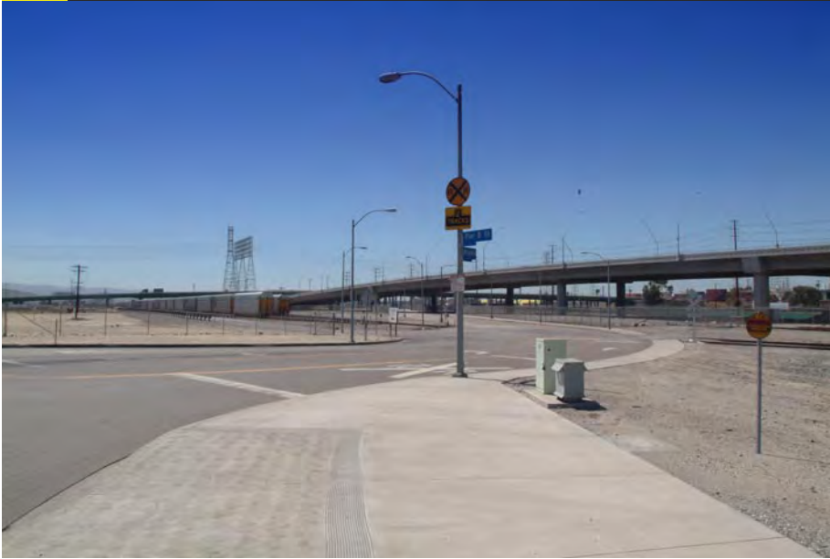
Anaheim Way at Pier B, looking northwest
