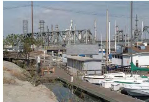
North side of East Basin Channel
