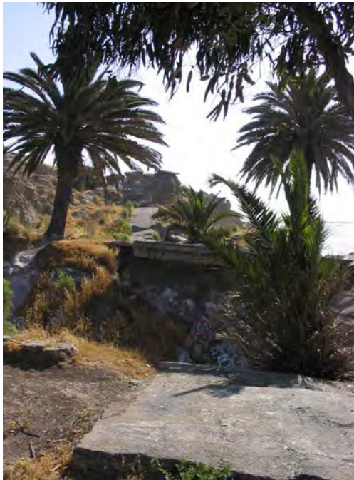
Former road in Sunken City
