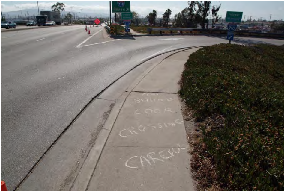
Anaheim at 710 Freeway, looking west
