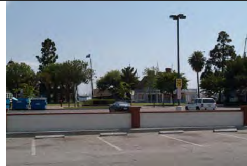
Half wall separating Timms Way from Ports O'Call
