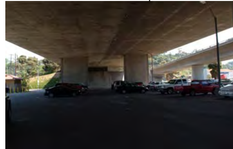
Parking lot under 110 freeway
