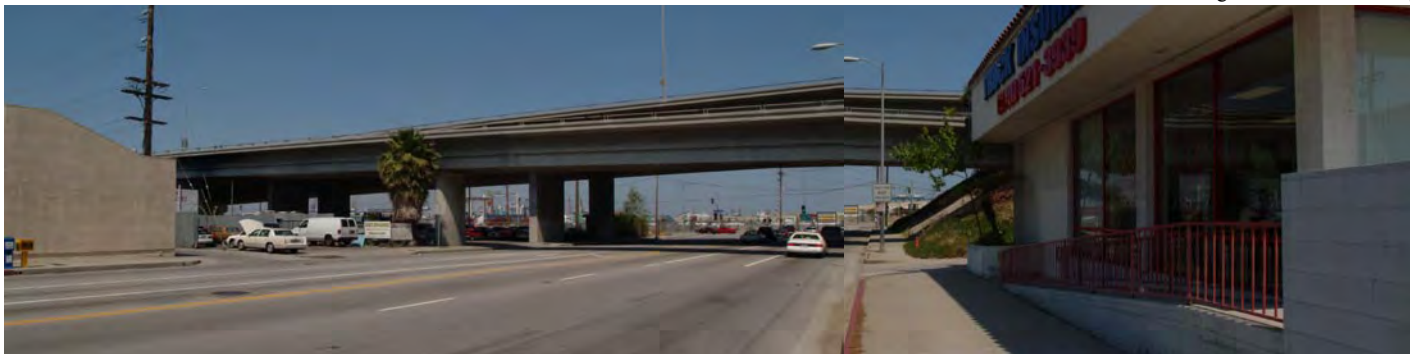
Channel at Gaffey panorama, looking east
