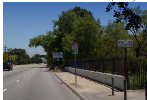
PCH at Wilmington Drain
