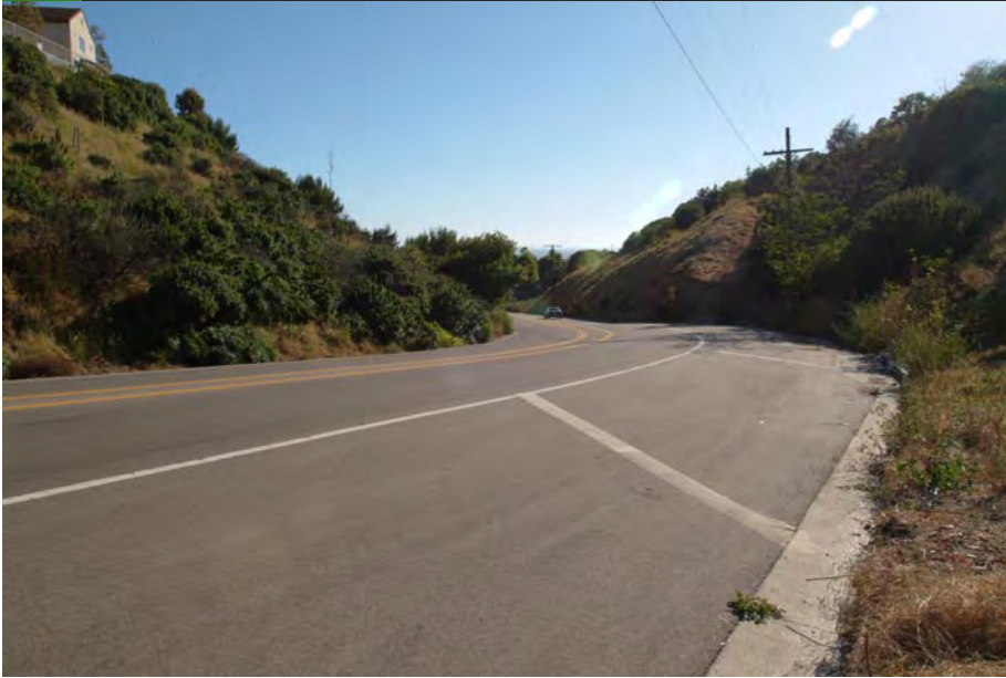
Western Avenue, looking south
