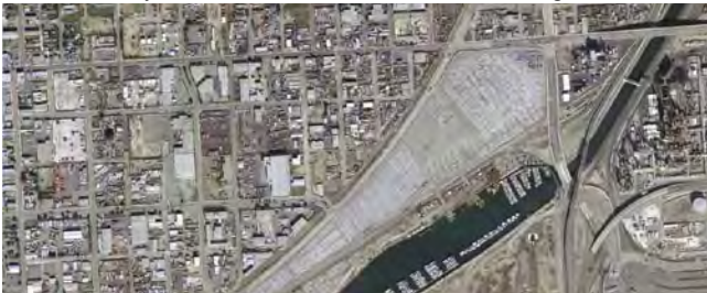
Aerial view of East Basin Channel
