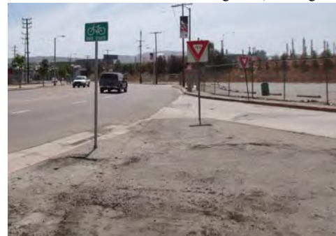
John Gibson at Figueroa, looking west
