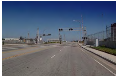
Pier A, looking east
